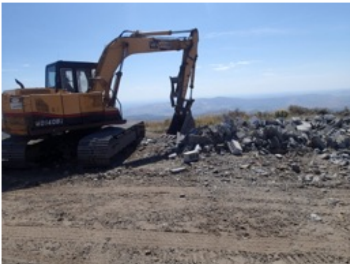
Demolition of the Bell Mountain Lookout (photo taken Oct. 16)
