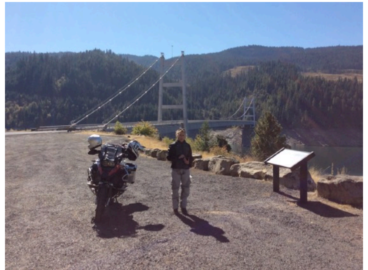
Looking South at the Dent Bridge over the Clearwater River.
