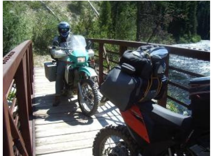
Bridge on beginning of Trail #021 at Deadwood Reservoir.
