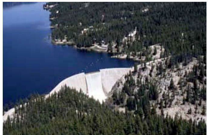
Aerial view of Deadwood Reservoir Dam on Deadwood River.
