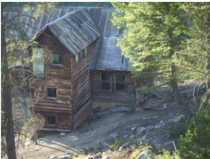
Old building (miner's barracks) at one of the mine sites north of Deadwood Reservoir that can be seen from the road (Landmark Stanley Road FS Road #579).
