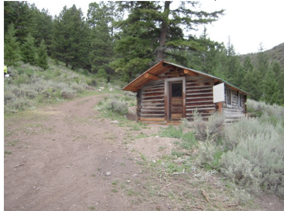
Site 4 area. Anderson Cabin is a restored typical miner cabin in the back area of the loop.
