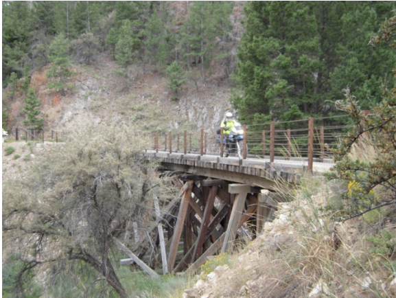
Site 18: Renovated Shay mining railroad trestle bridge.
