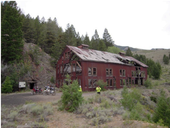
Air compressor facility at the Cossack Tunnel for operating the miner's tools and machinery
