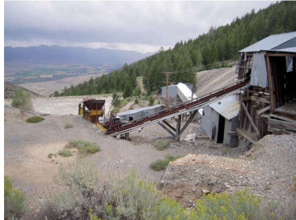
View of Empire Mill facing south.
