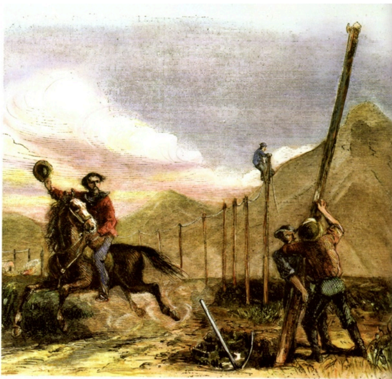
A Pony Express rider passes workers constructing the telegraph system that will eventually contribute to the demise of the legendary mail delivery system. (Courtesy of the Granger Collection.)
